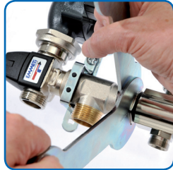
Fig. 5 Tightening the swivel joints
