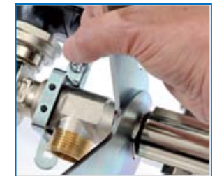
Fig. 3 Tightening the swivel joints
