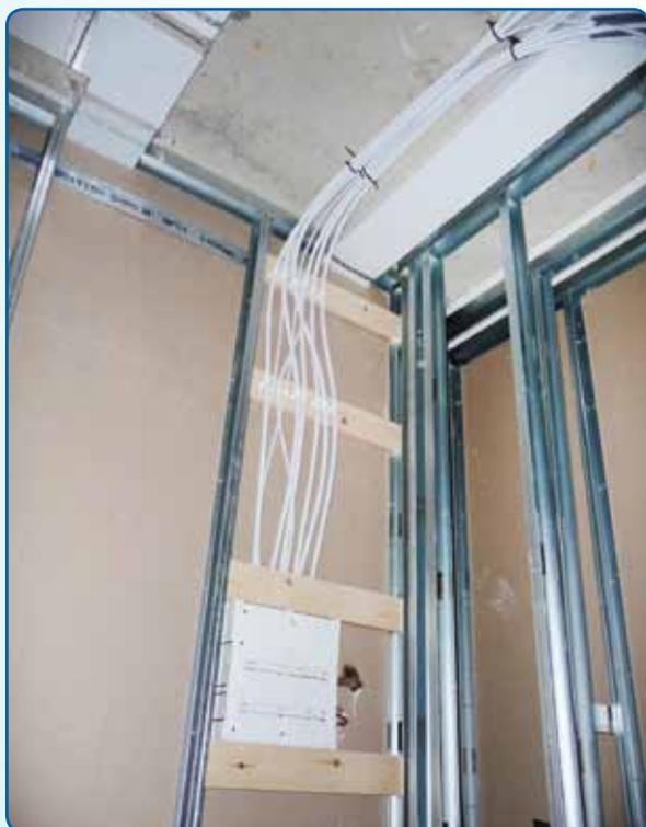
*The view from behind the plastic cabinet, this example shows the plasterboard now in place. Note the rising pipework and it's similarity to electrical wiring.*
