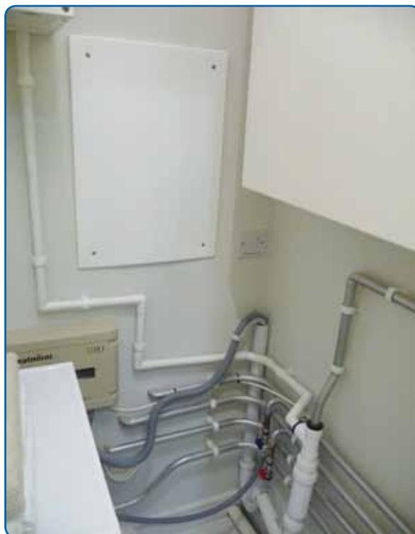
*The front of the cabinet, with the cover panel screwed down, concealing the manifold set. This is in a completed apartment installation.*
