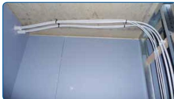
*A further example of suspended pipe bundles under the concrete plank construction.*
