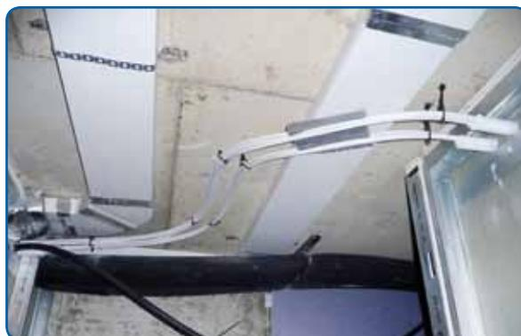
*This image illustrates the suspended tie cables keeping the pipes together and carrying their weight. Note the use of large diameter pipe to guide the bundle through a partition.*
