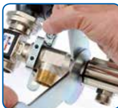
Fig. 5 Tightening the swivel joints
