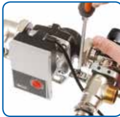
Fig. 4 Re-fit mounting bracket
