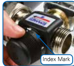
Fig. 10 Adjust the setting number against the index mark as shown
