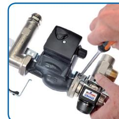
Fig. 3 Remove mounting bracket clips
