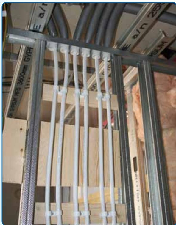
*The 15mm PB pipe rises up the inside of the metal stud wall, and goes into a plastic flexible conduit that is insulated. These isolated pipe run through the ceiling void and drop down to the terminal fittings.*
