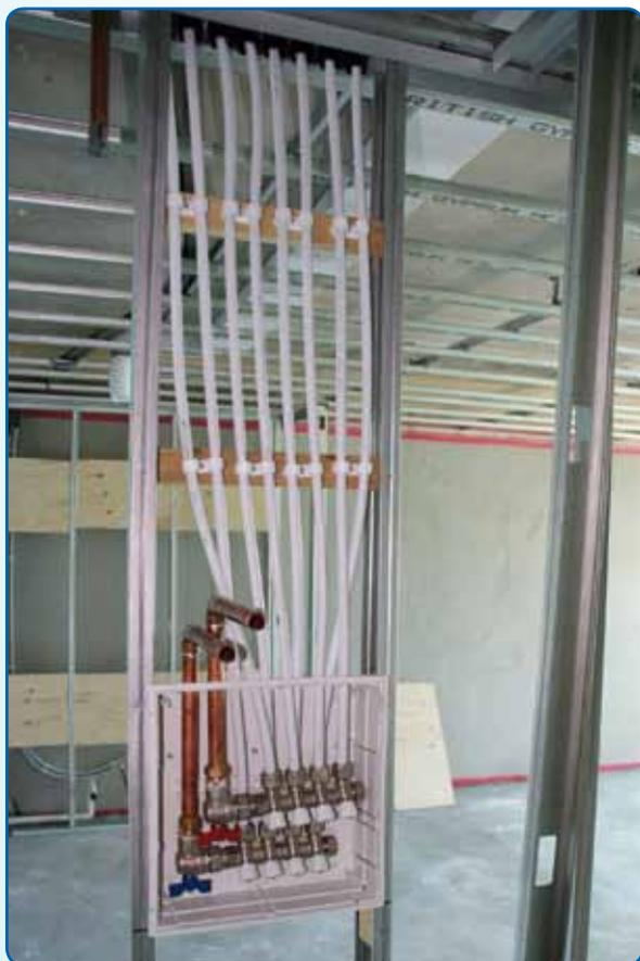
*A complete sanitary manifold set, the MULTIPLEX is shown here. This has been pressure tested and is ready to be plaster boarded in. Note the simple wooden battens used to support the pipe.*
