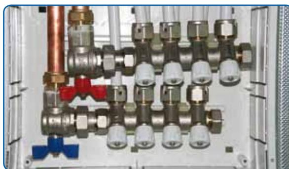
*Installed at first fix, the pair of elbow isolator ball valves help to isolate for pressure testing, and identify the hot and cold manifolds.*
