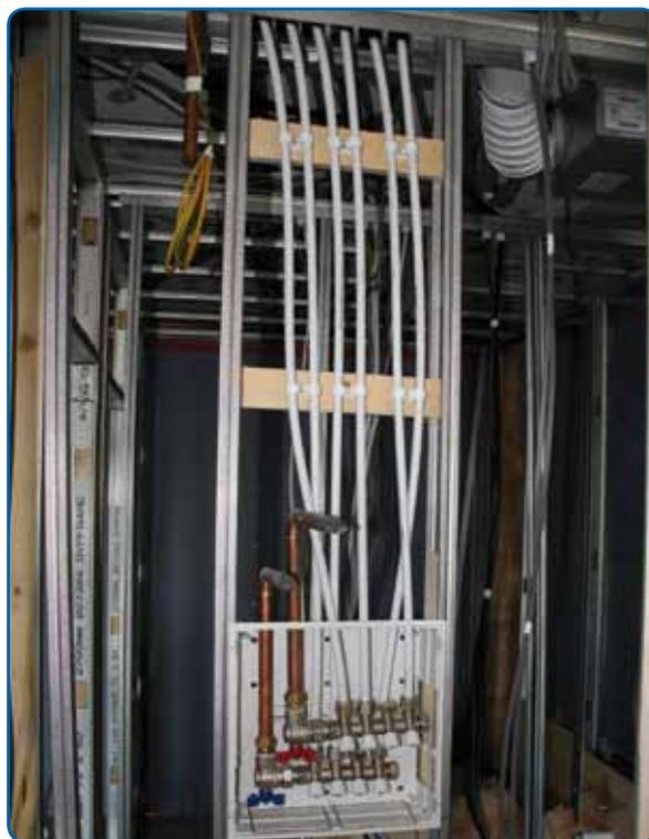
*The plastic housing cabinet is recessed directly into the metal stud wall. It has knock out panels to allow the pipe to rise out of the top.*
