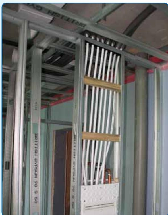
*The back of the plastic cabinet is flush with the metal stud wall. The two simple wooden battens support the pipe runs.*
